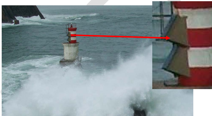
Figure 1 Entrance of Pasajes Port - Special bracket arrangement to protect the solar panel from wave force impact
