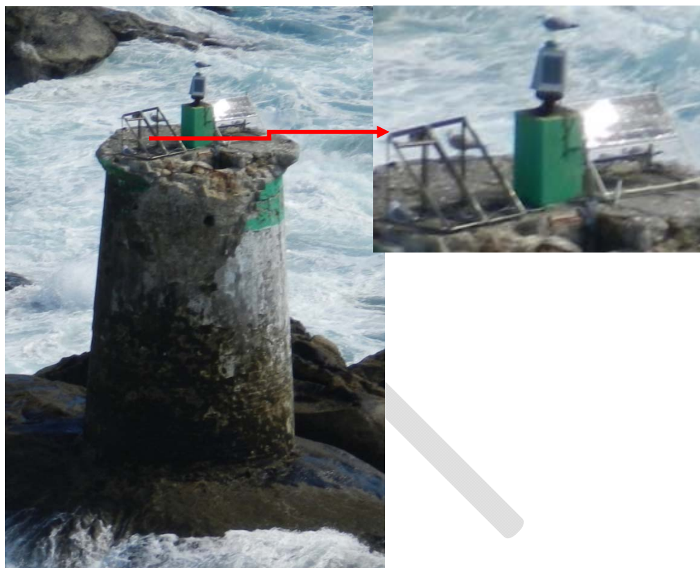
Figure 2 Northwest of Spain – Galicia coast – Structure and solar panels damages
